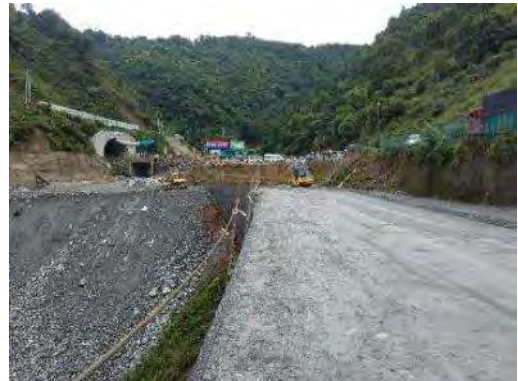
Visit to Approach Road (West Side)
