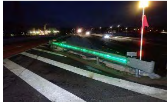
Nakdunga Tunnel Approach Road
