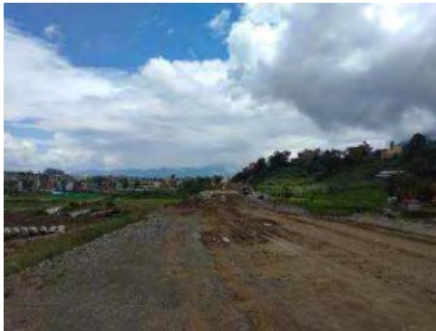
Approach road (east side) inspection
