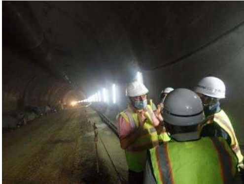
Visit to Nakdunga Tunnel
