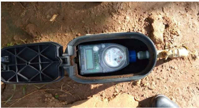
Typical Customer house connections in Lusaka
