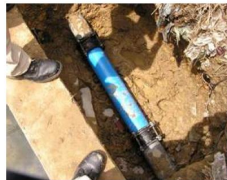
Leak repair by cutting and inserting a pipe piece using couplings
