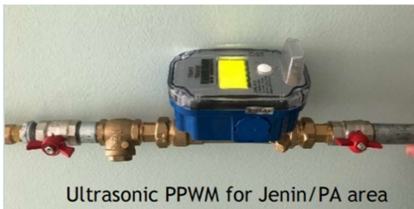
Ultrasonic type PPWM and fittings
