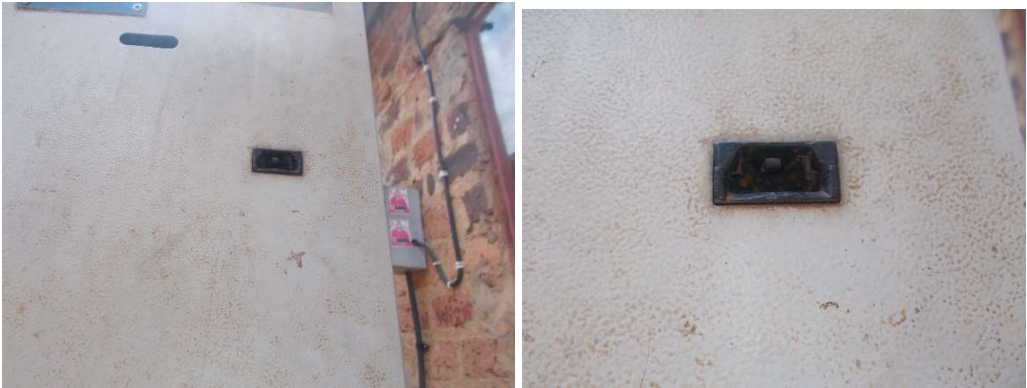
Vandalized public PPWM in Kampala
