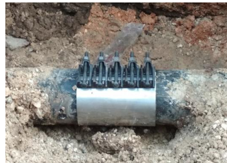
Leak repair by Repair clamp
