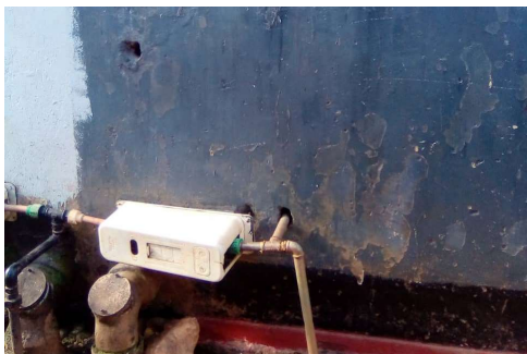
Protecting PPWM from water logging: Off the ground (left) and Wall installation (right) in Lusaka
