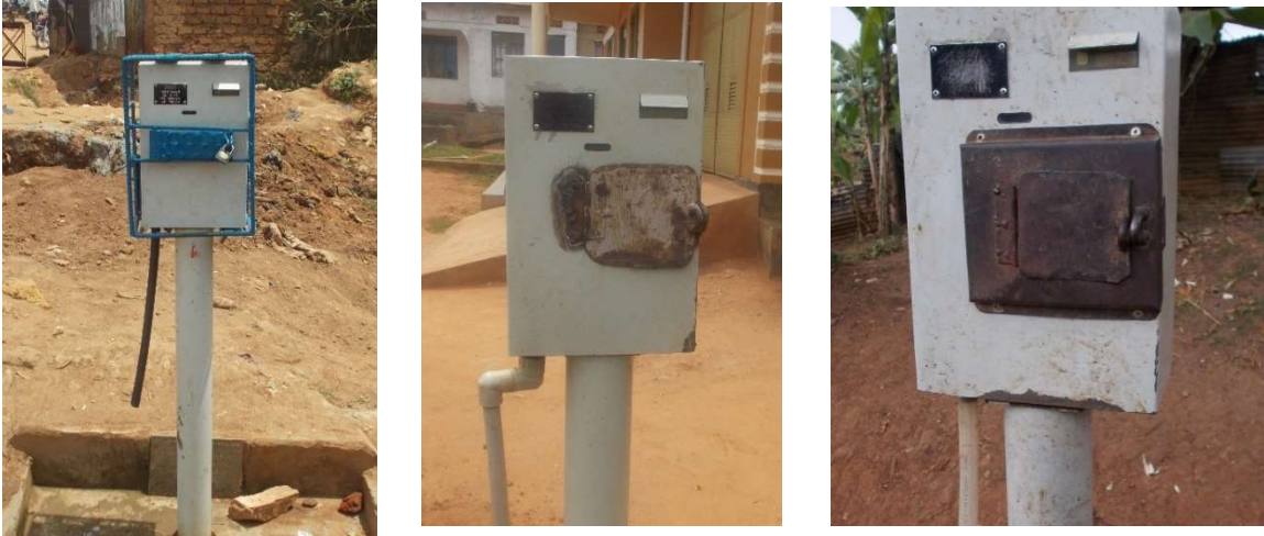
Photo 2 Improvisations for the protection of PPWM
