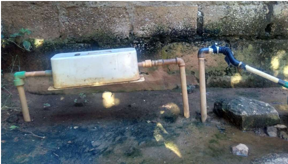
Protecting PPWM from water logging: Off the ground (left) and Wall installation (right) in Lusaka
