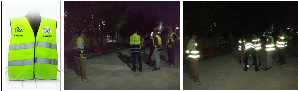
Figure 20-1: Uniform designed and used in this project (left), night time work (middle and right)
