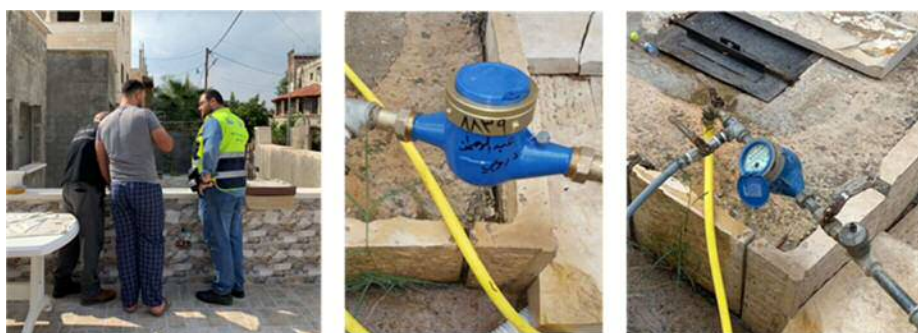
Photo 2-3 0-meter reading visit, broken meter and new meter after replacement
