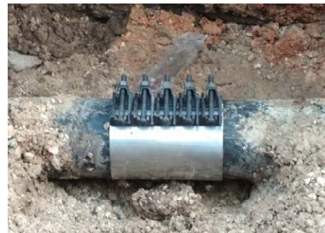
Leak repair by Repair clamp
