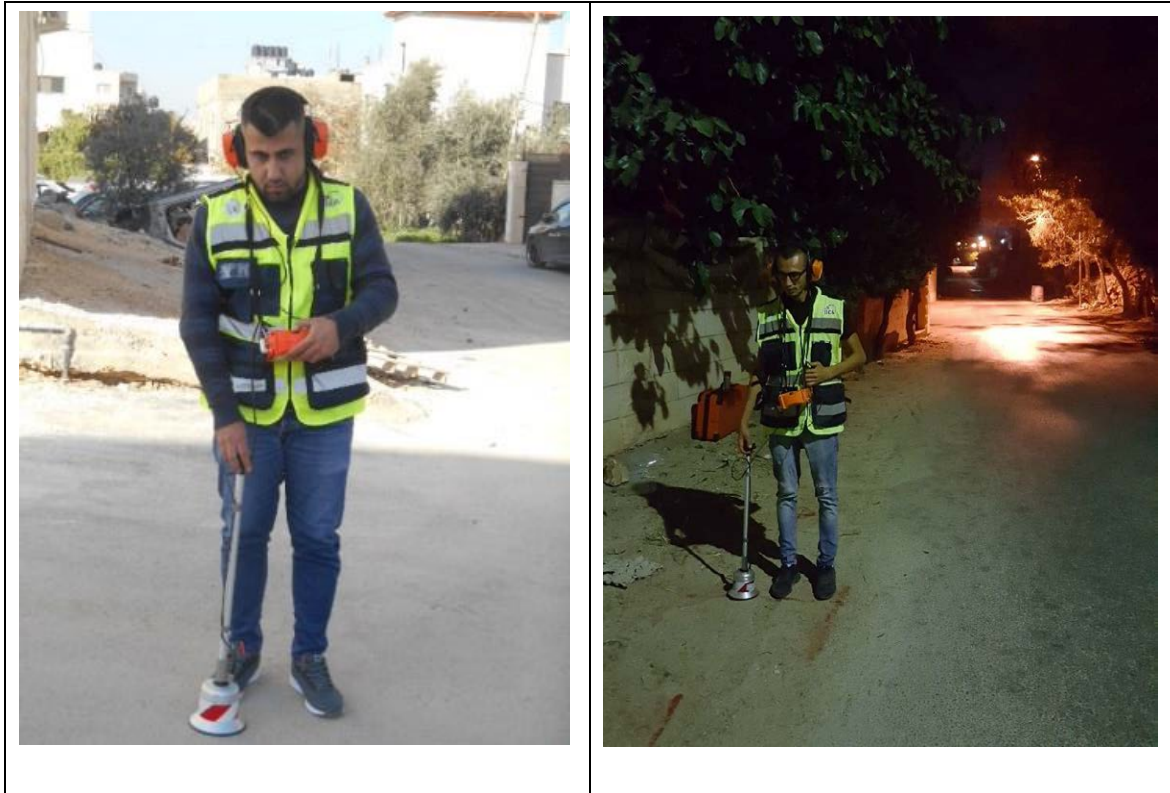
Figure 12-3: Line-Wise Survey Using Ground Microphone
