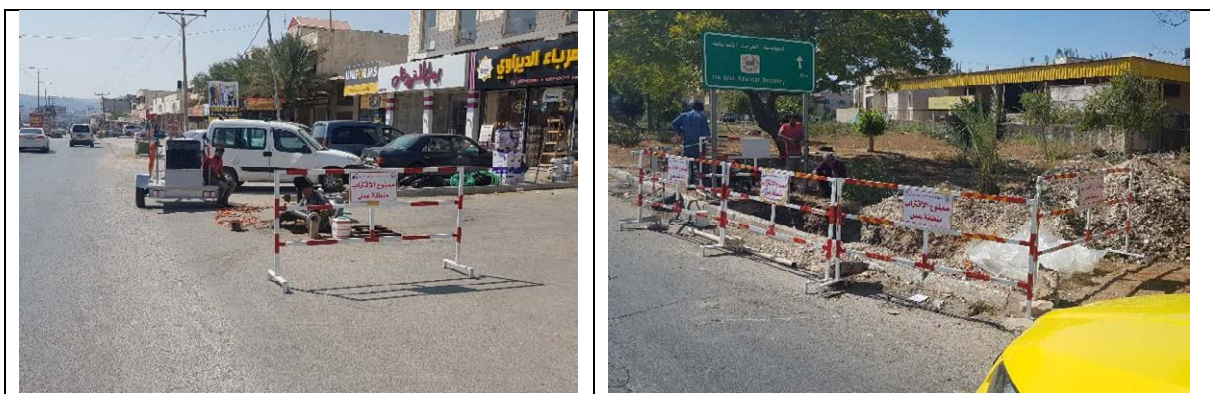
Figure 20-2: Barricade prepared and used in the project as a safety measure
