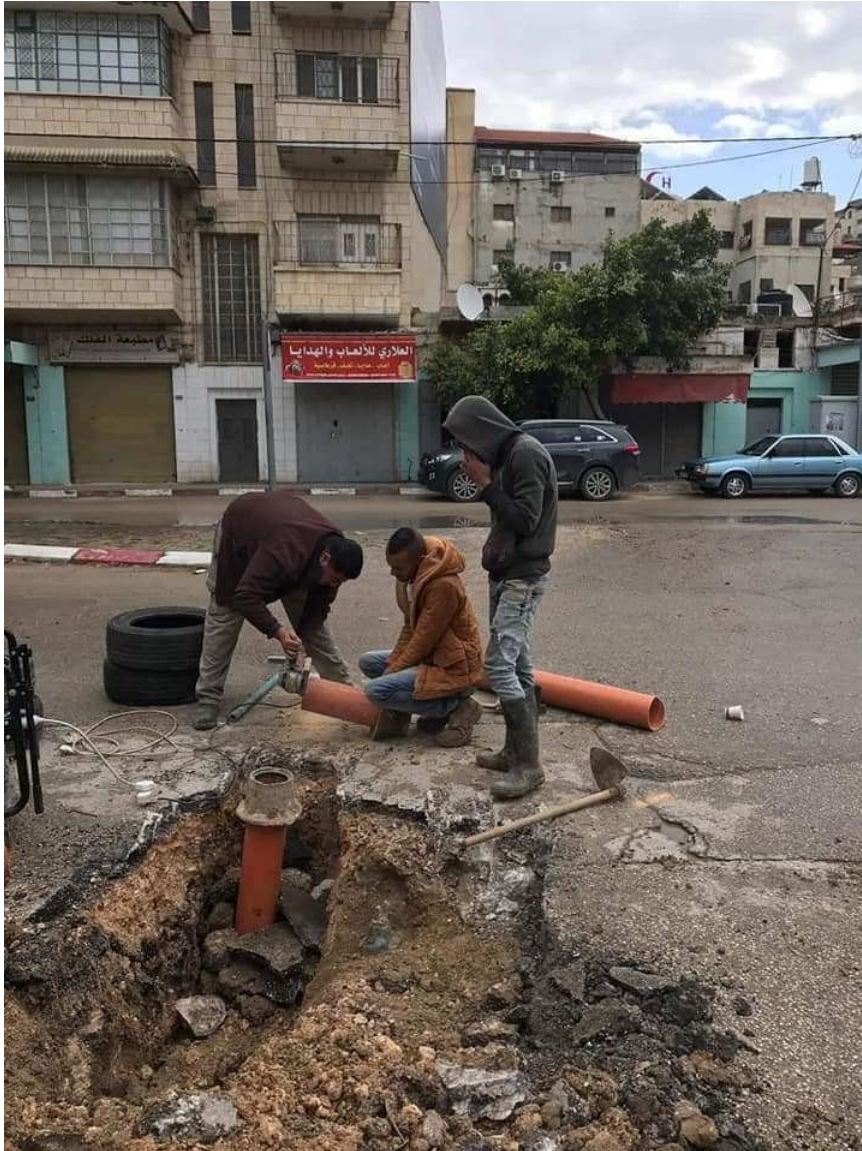
Cutting and Adjusting New Handhole Tube
