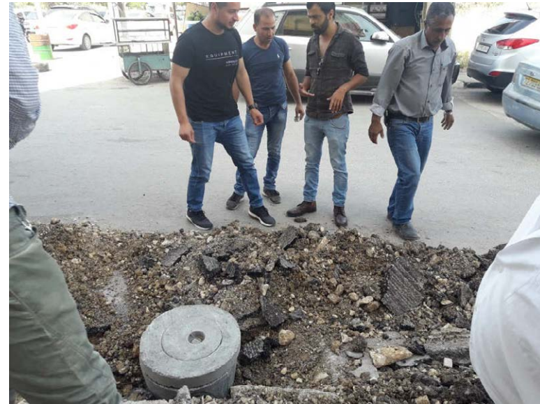
Excavate and expose 2" valve near Al-Nakheel building (valve opened)
