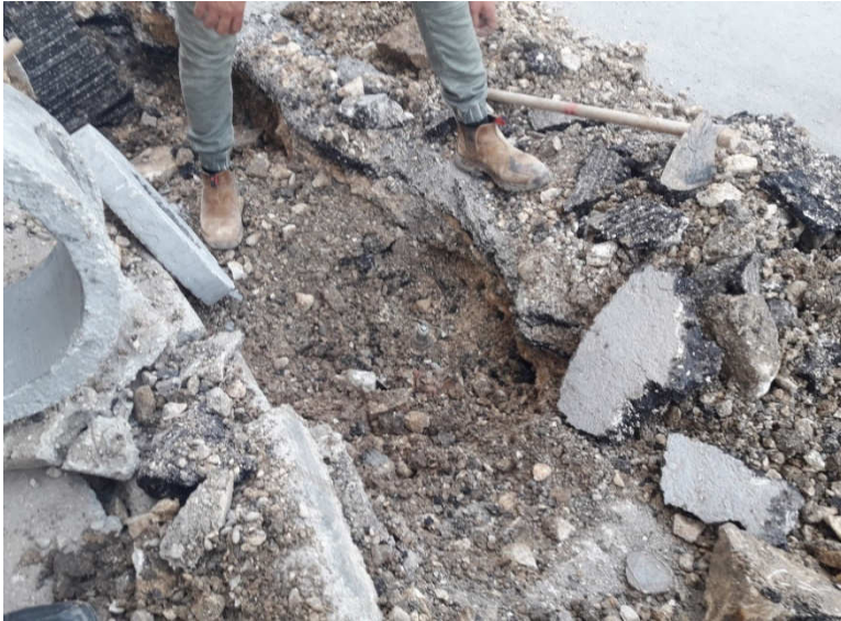
Excavate and expose 2" valve near Al-Nakheel building (valve opened)
