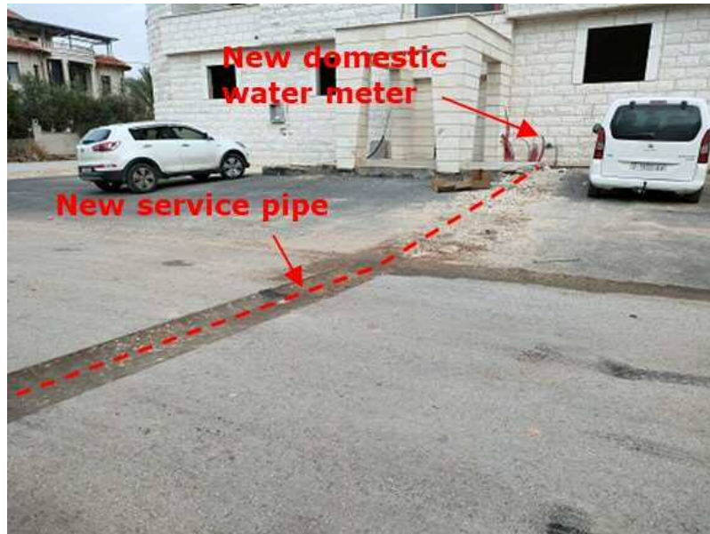
Photo 3.1 New service pipe installation
