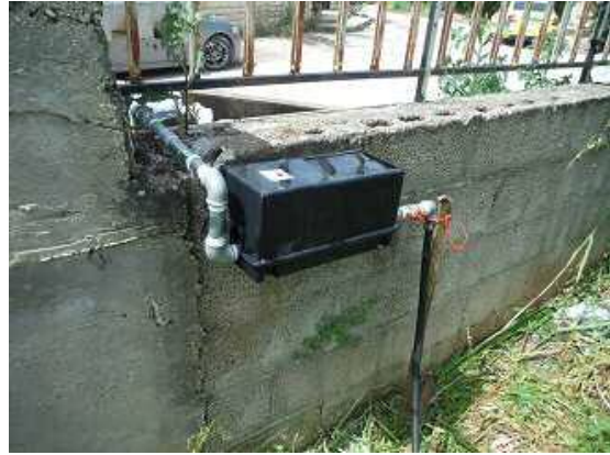
Photo 6.3 Horizontal installation
