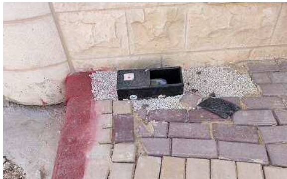
Photo 6.5 PPWM installed below ground level
