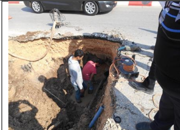
Photo 3.3 Digging for Leak Repair
