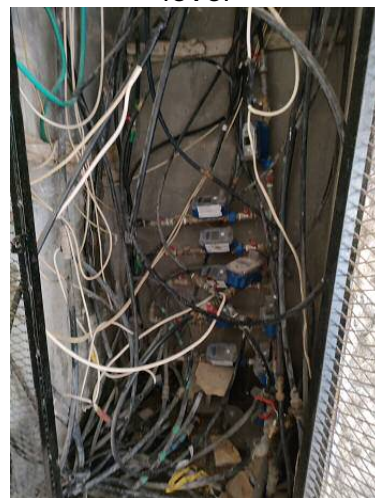
Photo 6.7 PPWMs installed in narrow space
