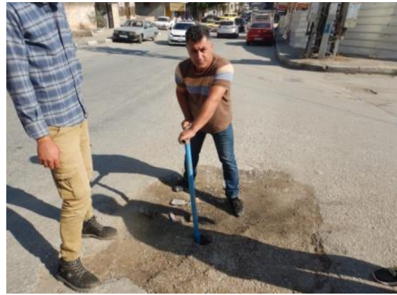
Photo 1.2 Valve Operation on a Street
