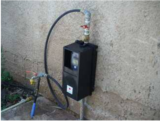
Photo 6.2 Vertical installation
