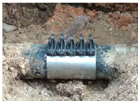
Leak repair by Repair clamp
