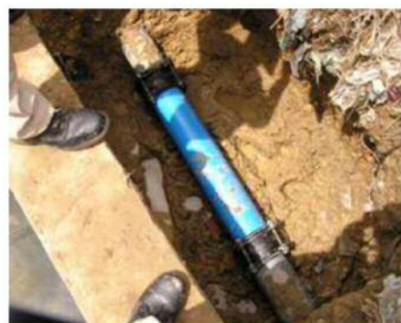
Leak repair by cutting and inserting a pipe piece using couplings
