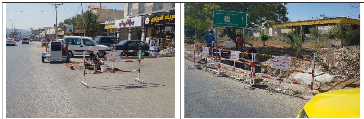
Figure 29: Barricade prepared and used in the project
