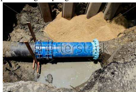
Repairing metallic pipe by flanged connector in one side and dismantling joint in another
