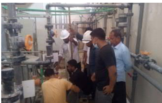
Photo 4. Training on chlorine injection equipment at the Karnaphuli water treatment plant (photo in March 2020, provided by the executing agency)
