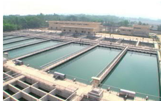
Photo 1. Karnaphuri water treatment plant constructed by the Project (a photo from JICA's project documents)
