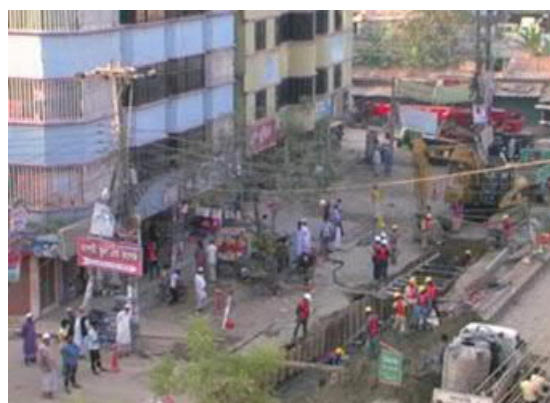
Photo 3. Work to lay distribution pipes (photo from JICA's project documents)
