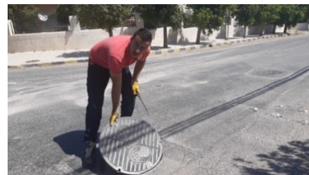
A YWC staff member distributing water by operating a gate valve in a manhole
