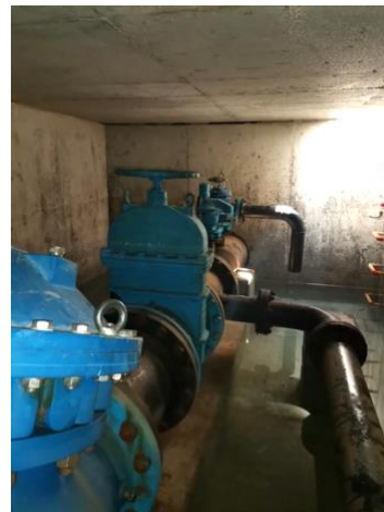
The distribution main and a pressure reducing valve installed by the Grant Aid Project
