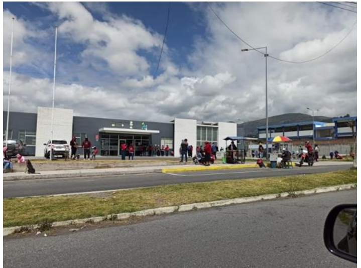
Carpi health center constructed under this project
