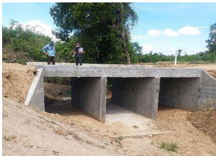
CMAC staff assisting bridge construction after demining activities
