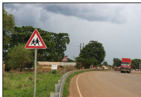
Installed guardrail and road sign
