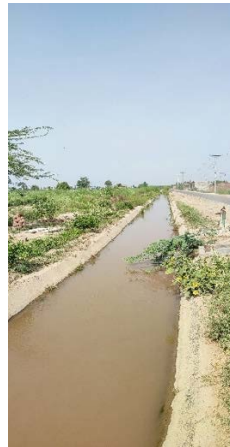
Figure 7. Good O&M Conditions at Padhyara Distributary
