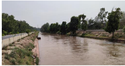
Distributary Rehabilitated by the Project
