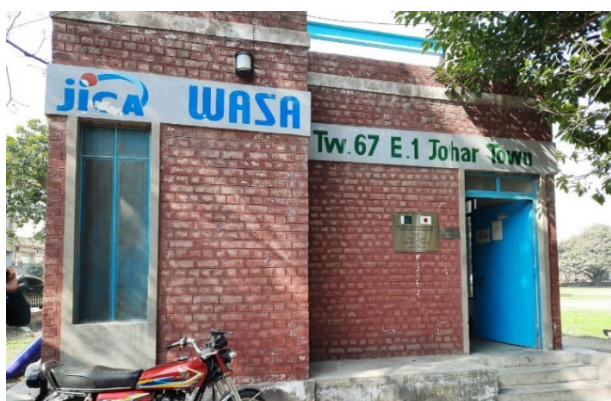
One of the tubewells constructed by the Project
