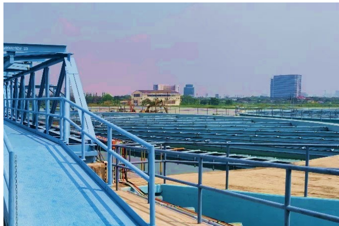
Bangkhen Water Treatment Plant
