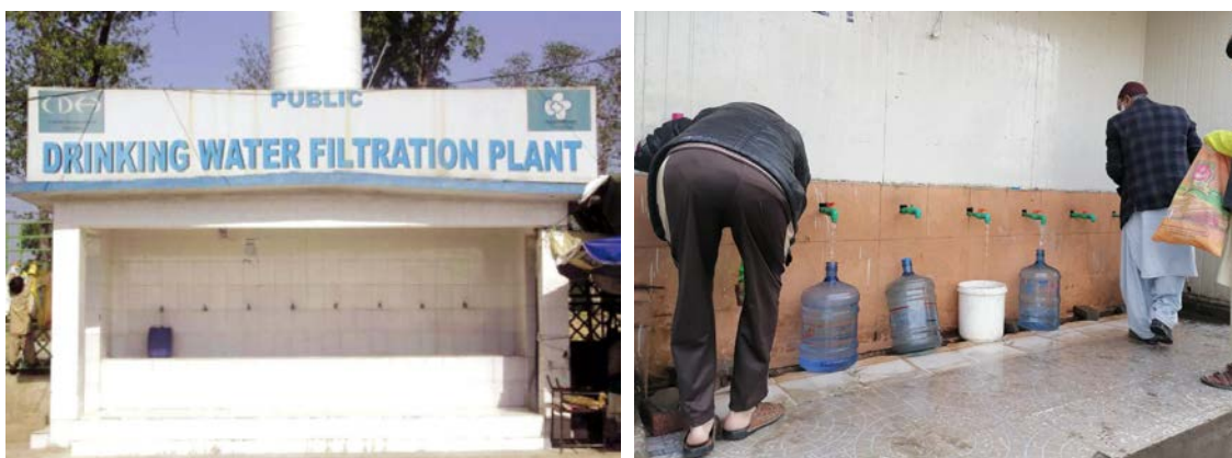
Arsenic removal facility constructed by the Pakistani side
