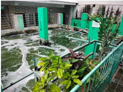
Photo 2 Wastewater treatment facility
