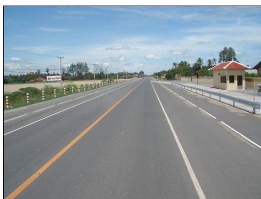
National Road No.1 (at the completion of Phase 3)
