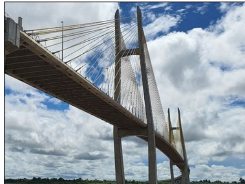
Neak Loeung Bridge
