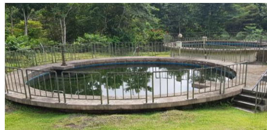
Vailima Water Treatment Plant
