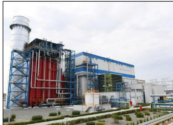
Shimal gas combined cycle power plant (Second unit)
