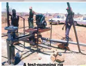
A test-pumping rig
