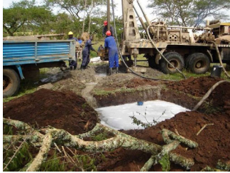
Mud Drilling and Location of Mud Pit
