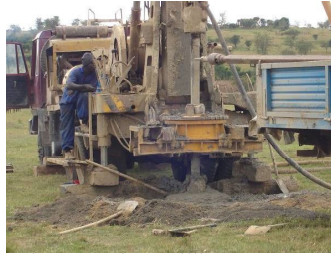
Air Percussion Drilling
