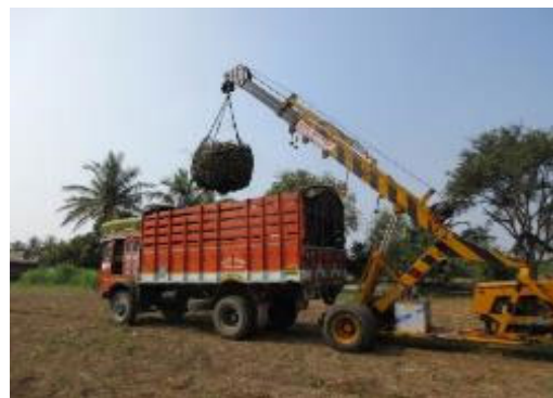
Loading (Mobile Crane to Truck)
