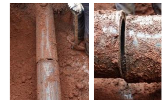
Disconnection of HDPE Pipes by water pressure test
