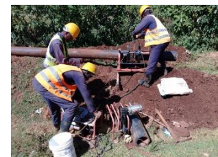
Butt fusion method
