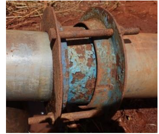
Repaired by VJ Joint
