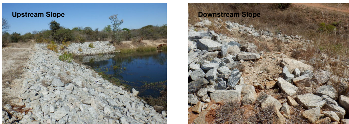
Figure 5.3.72 Upstream and Downstream Slope
