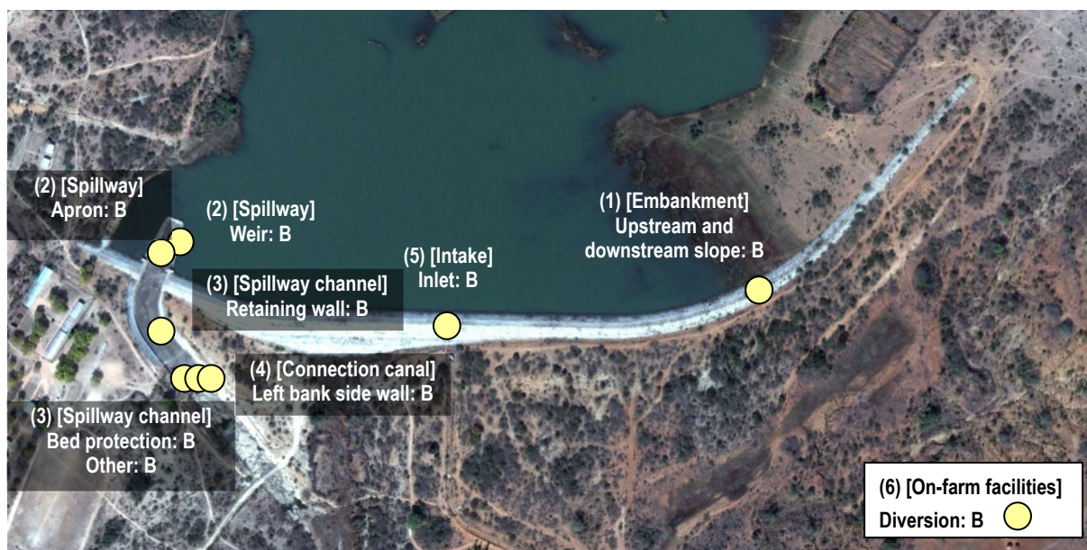
Figure 5.3.68 Locations of Deteriorations/Damages on Munjanganja Dam
