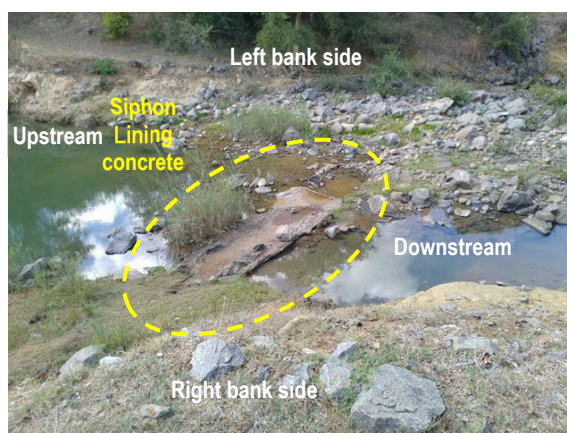
Figure 5.3.11 Exposure of Siphon Lining Concrete
