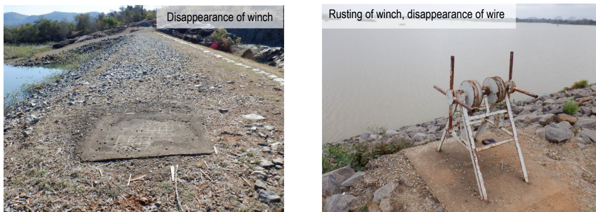
Figure 5.5.18 Status of Intake Structures
