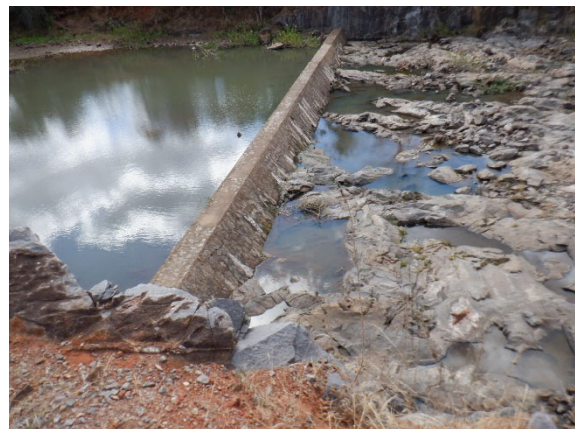
Figure 5.3.7 Panoramic View of Weir
