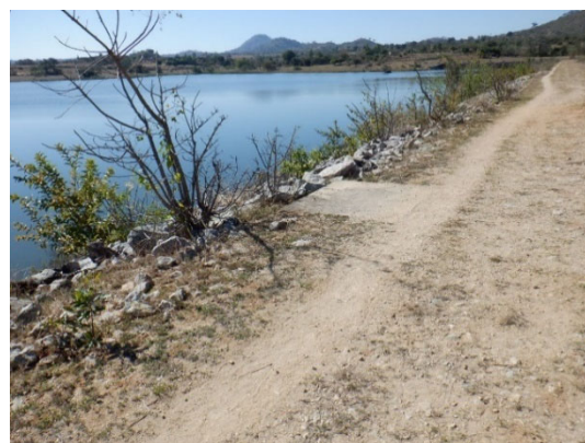
Figure 5.3.45 Disappearance of the Intake Gate Operation Facilities
