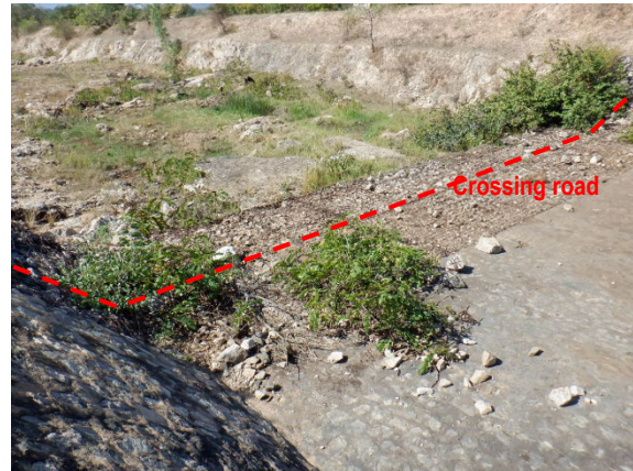
Figure 5.3.55 Crossing Road across the Channel
