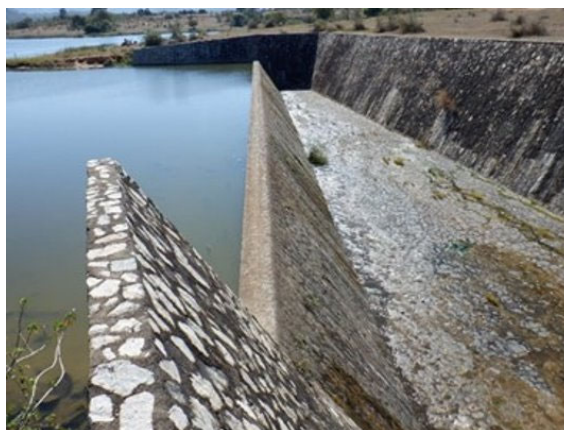
Figure 5.3.40 Panoramic View of Weir
