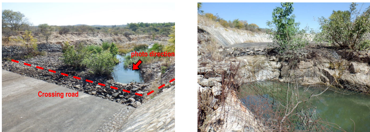
Figure 5.3.76 Spilling Out of Basket Mat at the Right Bank Side
