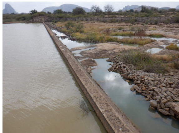
Figure 5.3.25 Panoramic View of Weir
