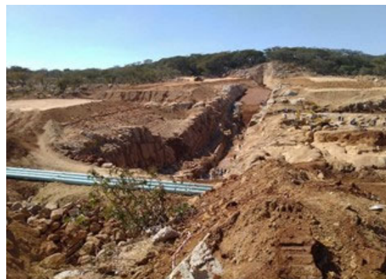
Figure 5.4.7 Construction Site of Chivu Dam
