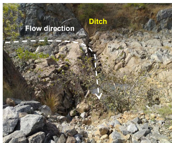
Figure 5.3.10 Suspected Reason of Collapses on the Right Bank Side (Embankment Side) Wall
