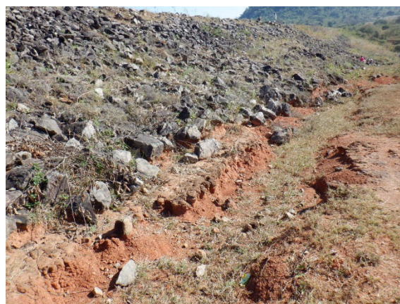
Figure 5.3.65 Downstream Slope Edge
