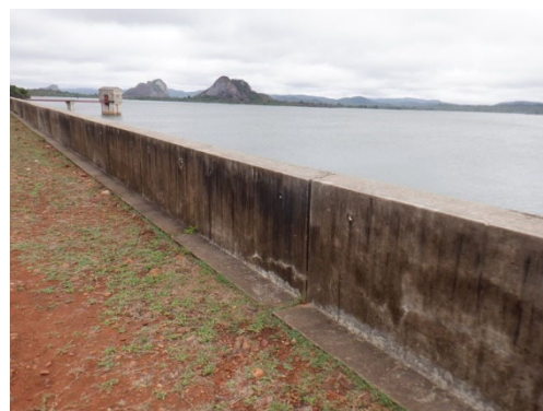
Figure 5.5.10 Example of Parapets (Mundi Mataga Dam)
