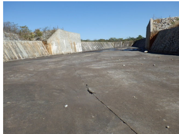
Figure 5.3.74 Joints of the Apron
