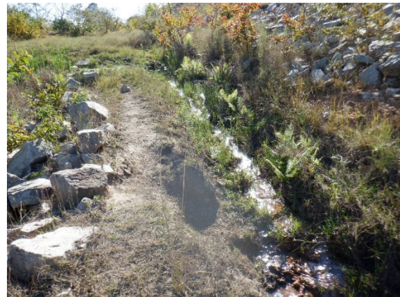
Figure 5.3.39 Downstream Slope Edge of the Right Side Abutment
