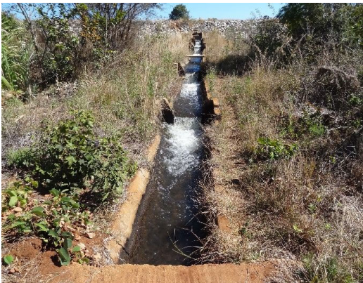
Good condition. OF(5):On farm canal(1)
