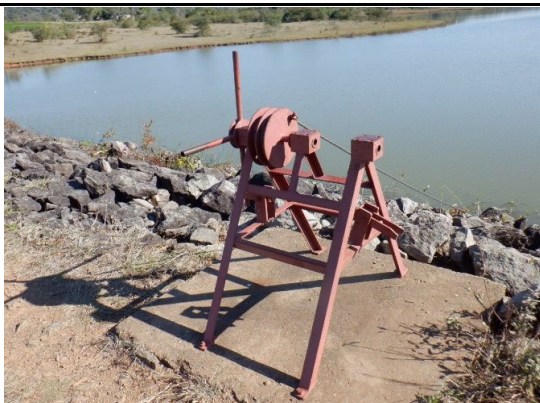
I(1) Intake Inlet: No significant damage is observed.
