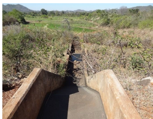
Good condition. OF(4):Night storage(Spillway)
