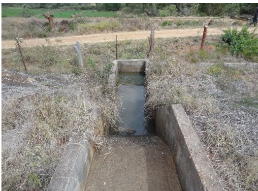
Good condition. OF(5):Night strage(Spillway)
