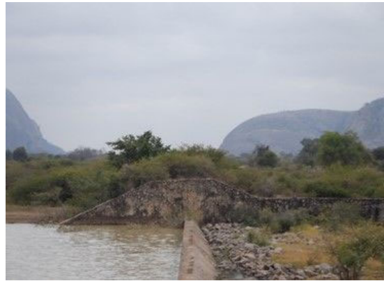
S(6) Spillway retaining wall (left): No significant damage.
