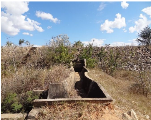
Good condition. OF(5):Night strage (Distribution facility)
