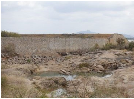
S(5) Spillway retaining wal (right)!: No significant damage.
