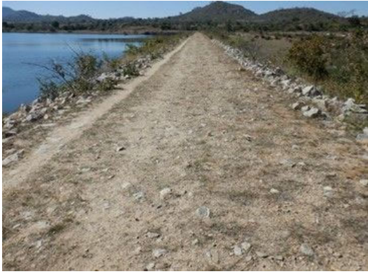
D(7) Crest of Embankment: Since no significant damage is observed.
