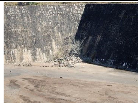
S(6) Spillway Apron: Stones are deposited at the upstream end.
