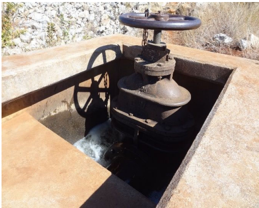
The valve is movable and in good condition. OF(3):Night storage(Outlet valve)
