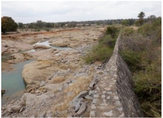
S(8) Spillway apron: The bed is digged rock. No significant damage.
