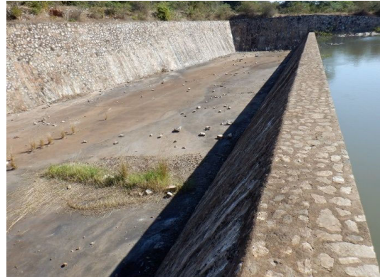
S(2) Spillway crest: No significant damage.
