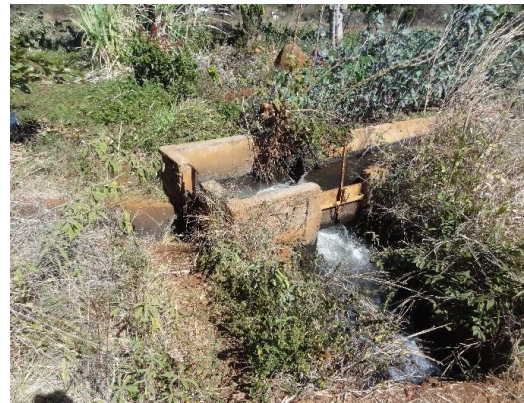
Good condition. OF(6):Diversion(1)
