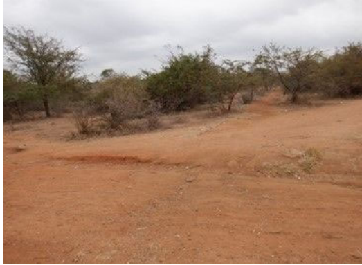
D(7) Right side abutment: No significant damage. Abutment area around edge of crest is flat.
