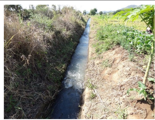
Good condition. OF(6):On farm canal(2)
