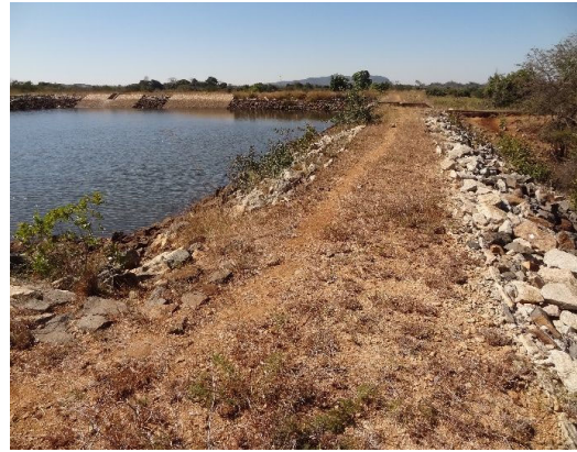
No sedimentation and good condition. OF(2):Night storage(2)
