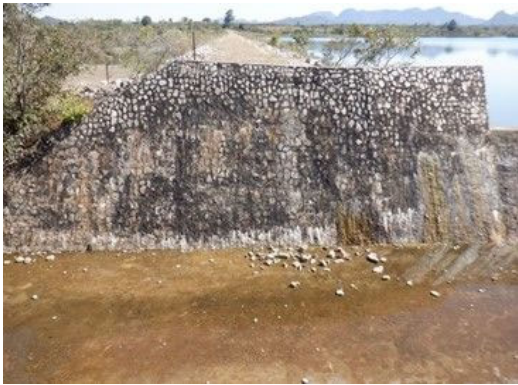
S(5) Spillway Retaining walls(right): No significant damages are observed.
