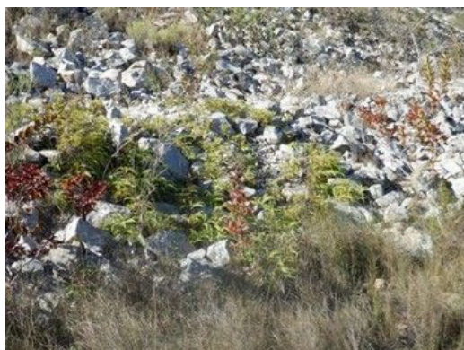
D(6) Embankment Downstream: Seepage and slight flow at the downstream slope edge. Around here, there are parts where the plants are different from those around them.
