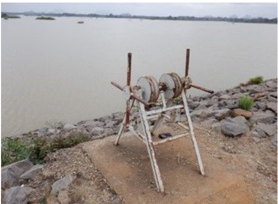
I(1) Intake Inlet:The winch is still in place, but the wires are disappeared. There is rusting all over. The handle on the right bank side is movable.
