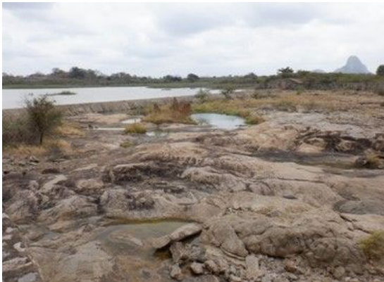
S(7) Spillway apron: The bed is digged rock. No significant damage.
