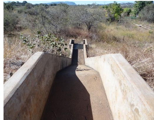
Good condition. OF(4):Night storage(Spillway)
