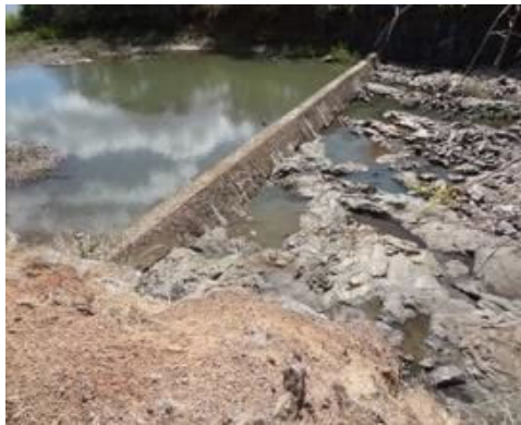
S(1) Spillway entire: No significant damage is observed.
