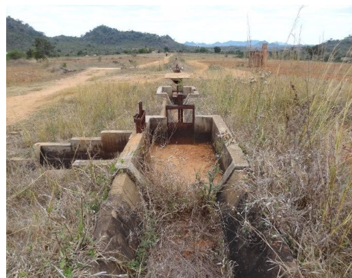
Good condition of movable gate and divirsion. OF(6):Diversion
