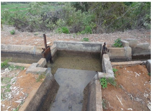
Good condition. OF(6):Diversion(1)
