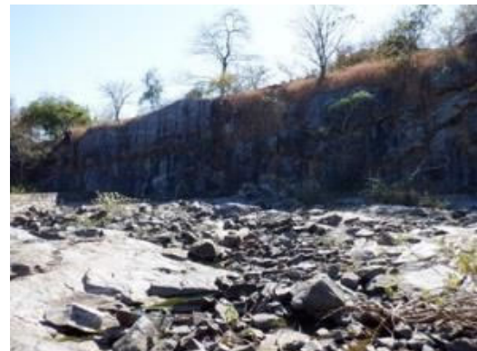
S(6) Spillway Retaining wall(Left side): No significant damage is observed.
