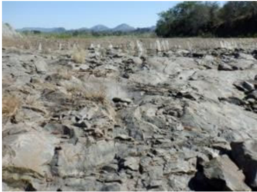
S(7) Spillway Apron: No significant damage is observed.
