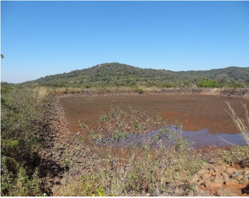
No sedimentation and good condition. OF(1):Night strage ( 1 )
