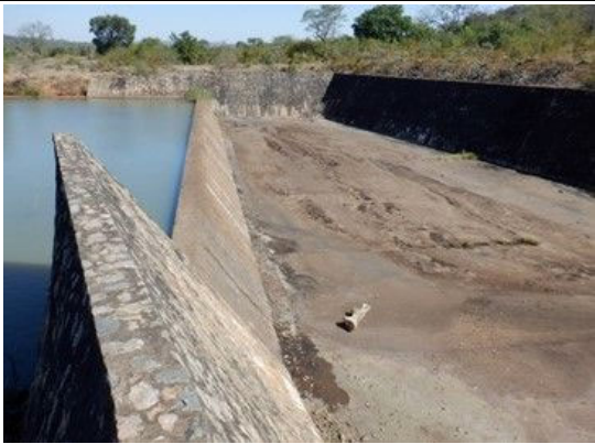
S(1) Spillway entire: No significant damage is observed.
