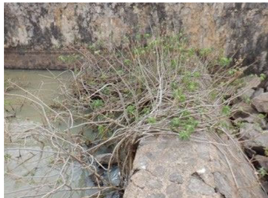
S(4) Spillway weir: A slight plants on the left bank side
