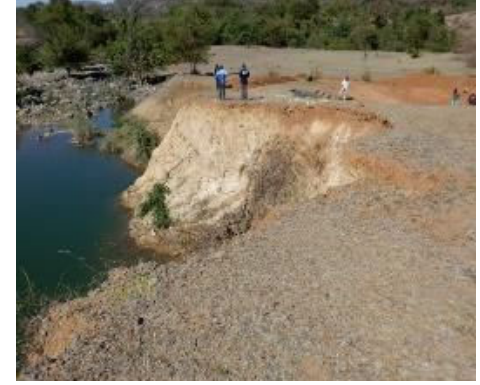
C(8) Connecting Canal:
