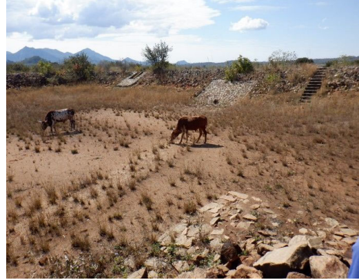
No sedimentation and good condition. OF(2):Night storage(2)
