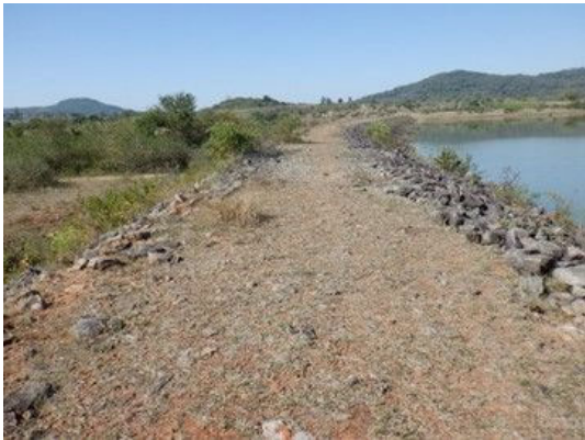
D(9) Crest of Embankment: No significant damage is observed.
