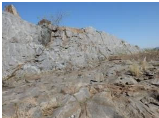
S(5) Spillway Retaining wall(Right side): No significant damage is observed.
