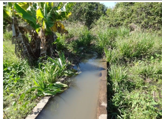
The end of the on farm canal is blocked by soil embankment. OF(12):On farm canal(6)
