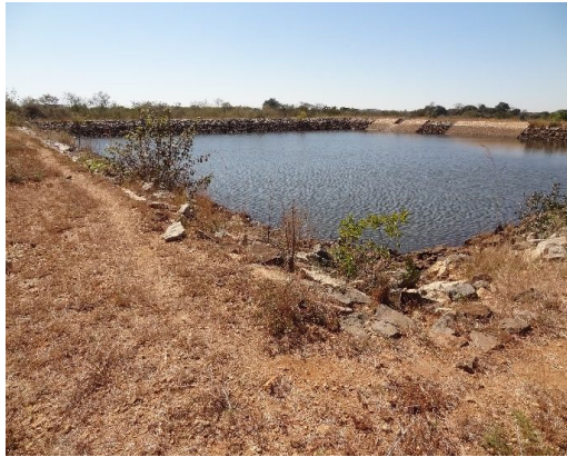
No sedimentation and good condition. OF(1):Night storage (1)
