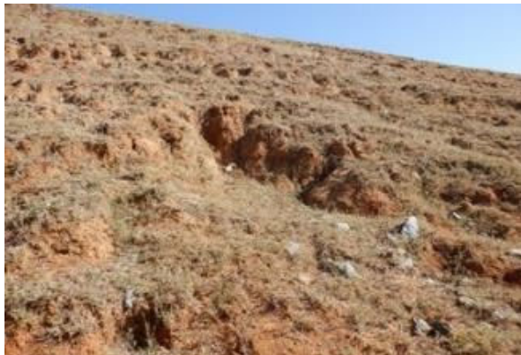
D(3) Embankment Downstream: Erosion depth about 80cm, depression depth 1.8m, width 2.7m, etc.
