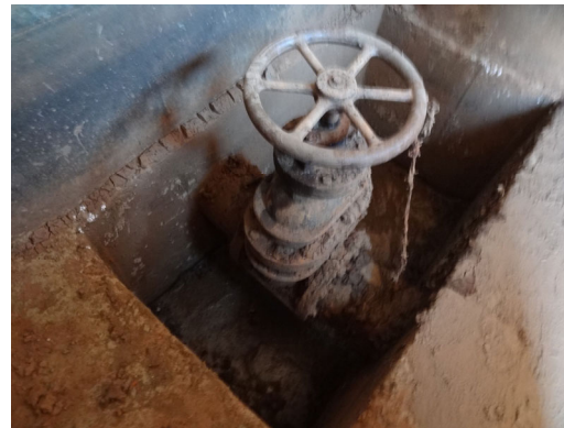
I(2):Outlet (Valve):Good condition.
