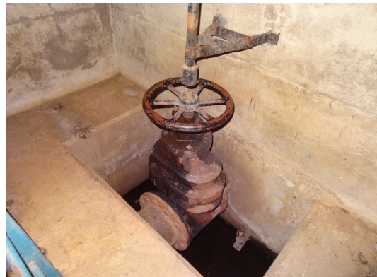
I(4) Intake Outlet: The valve has been controlled in good condition.
