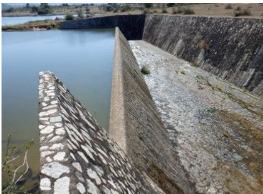
S(1) Spillway entire: No significant damages are observed.
