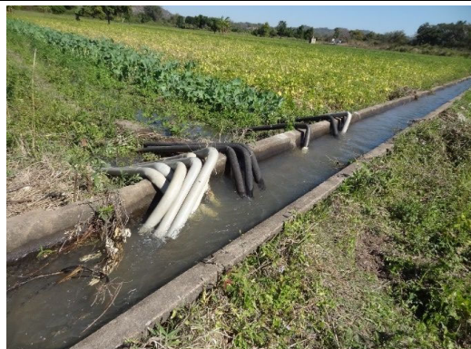
The water intake pipe from the on farm canal. OF(11):On farm canal(5)
