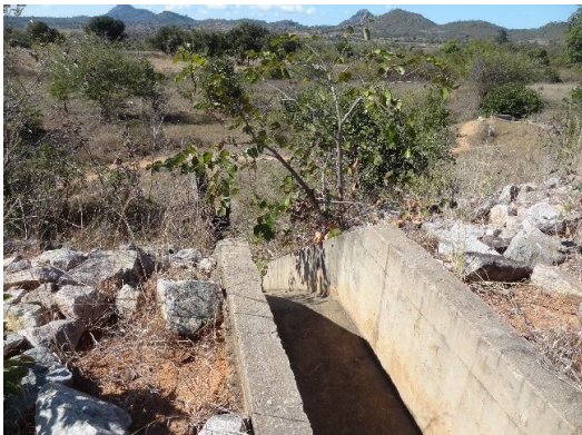
Good condition. OF(3):Night storage (Spillway)
