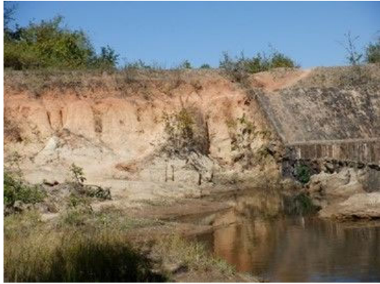
C(1) Connecting Cana(right): No significant damage is observed.
