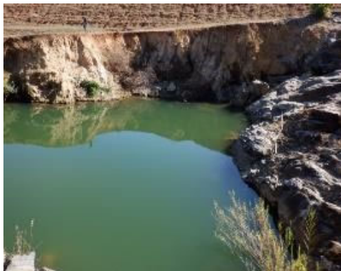
C(3) Connecting Canal: The large erosion is observed on the right bank side (embankment side).
