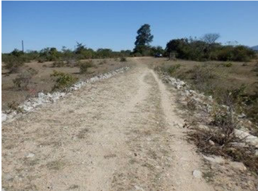
D(9) Right side abutment: No significant damages are observed. Elevation difference is small (hill-like terrain) .
