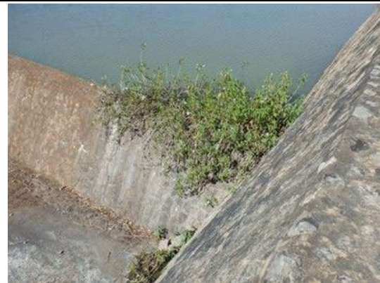
S(4) Spillway weir: Slight plants on the left side of weir.
