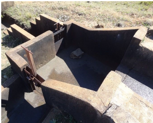
Good condition. OF(5):Night storage (Distribution facility)
