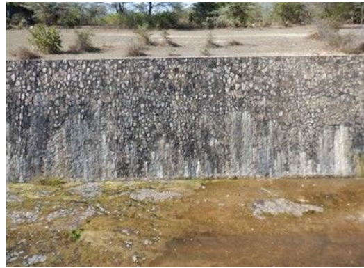
S(6) Spillway Retaining walls(left): No significant damages are observed.
