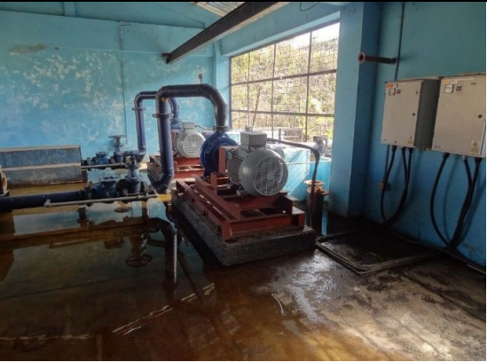
Electric pump equipment has been installed by FAO in 2016.
