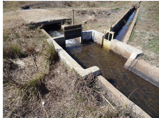
The diversion has been rehabilitated by FAO in 2019.
