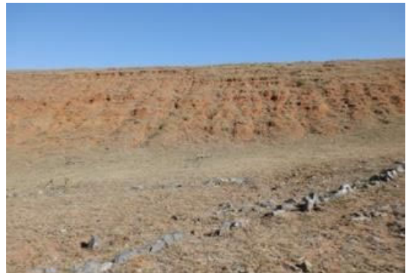
D(2) Embankment Downstream: Gully erosion on the downstream surface. A surface water flow path (ditch) has been created in the downstream direction.
