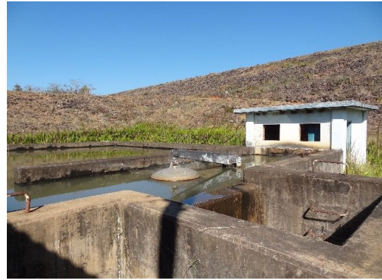
Rusted float valve
