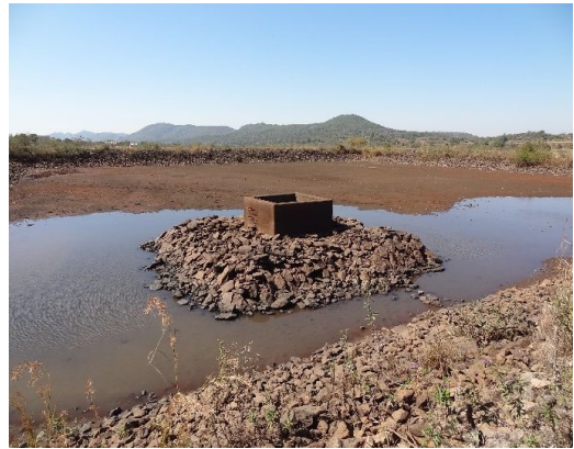
No sedimentation and good condition. OF(2):Night storage(2)
