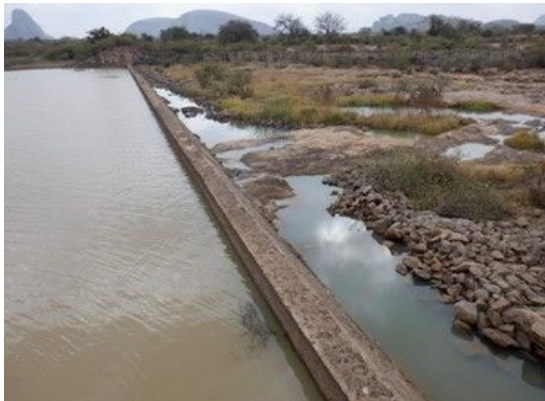
S(1) Spillway Entire: No significant damage.
