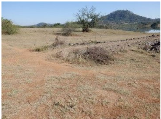
D(11) Right side abutment: No significant damage is observed. The abutment around the edge of the crest is flat.
