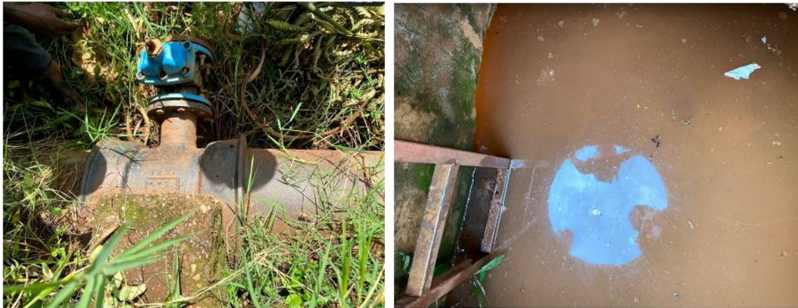
Photo (Left) Karengwe 1 pipe at Nyakaliro-Masaka boundary (Right) Leakage of Karengwe 1 or Karengwe 2 observed at a airvalve chamber
