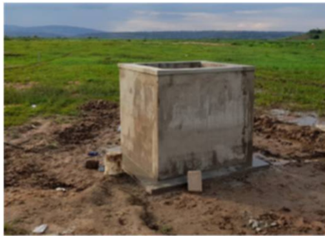
Figure 3-18 Protection of Well against Flooding
