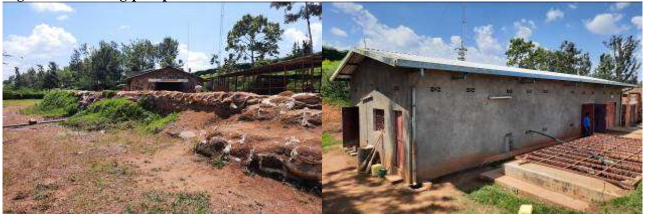
Figure 5: Existing pump house at intake
