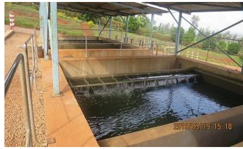
Rapid sand filters (3 series, 2 basins/series)
