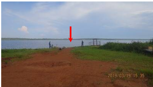
Water source and intake (center of the Lake, app. 500m from the Lakeshore edge) for Karenge WTP.
