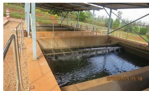
Rapid sand filters (3 series, 2 basins/series)
