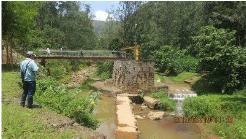
Intake for Kimisagara WTP
