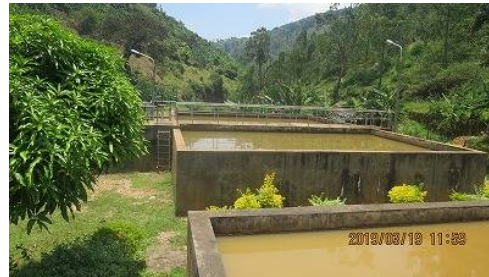
Pre-sedimentation tanks
