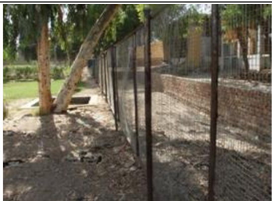
Photo 2-1 Wire-netting fence model, 2m High
