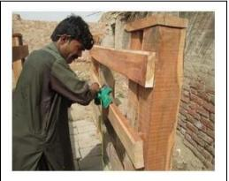
A carpenter cuts an edge of a rectangular timber using an electric plane
