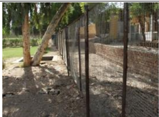
Photo 2-1 Wire-netting fence model, 2m High
