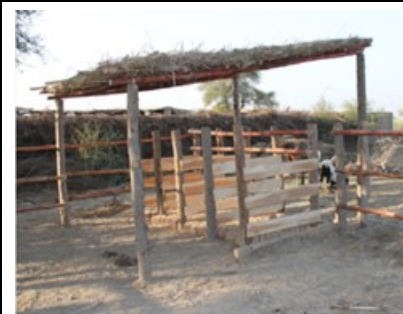
Photo 3-38 Roof with good ventilation
