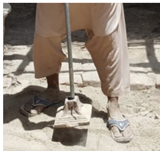
Photo 2-24 Tools for floor preparation
