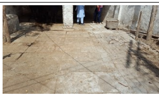
Photo 2-26 Floor after improvement
