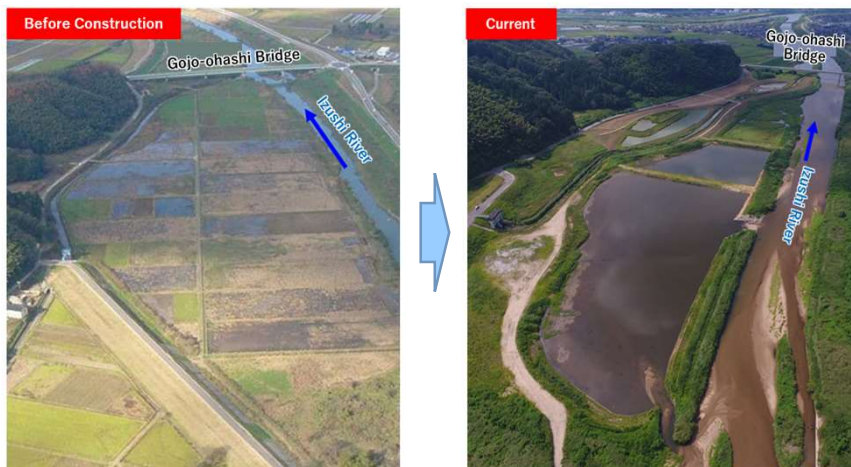
Source: MLIT Kinki Regional Development Bureau Toyooka River National Highway Office Website
