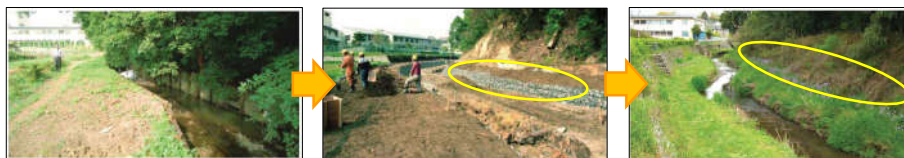
Before construction: plank hurdle revetment
