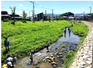
Green Infrastructure, Kamisaigo River Source: Fukutsu City
