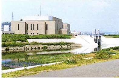
Internal Drainage Facility (Pumping Station)
