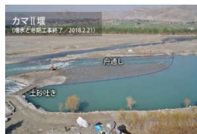
Kama II Weir (Afghanistan)
