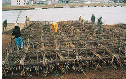
Riverbed and Riverbank Protection (Fascine Mattress)
