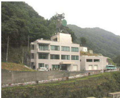
Source: Website of Tone River Dams Integrated Management Office
