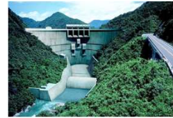
Source: Japan Dam Foundation
