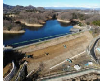
Seismic Resistance Reinforcing Works for Sannako Dam
