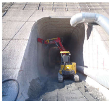
Source: Sendai-gawa River Office, MLIT
