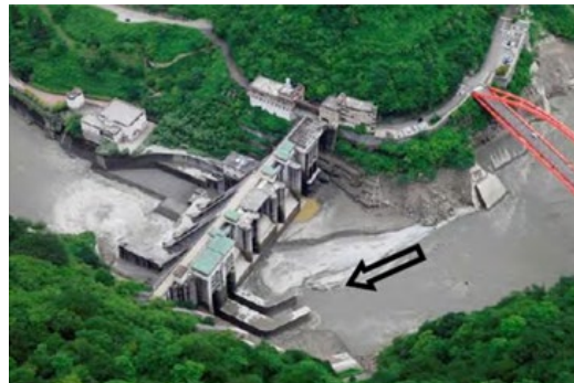
Flushing through sediment gates
