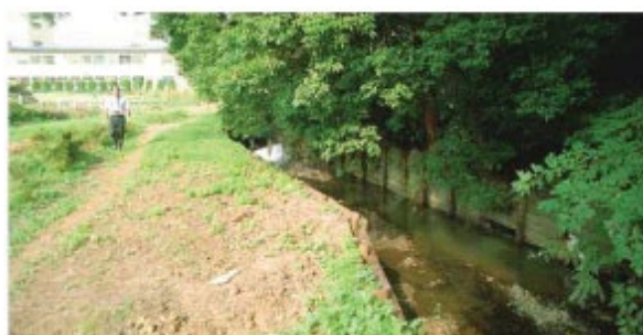
Before construction: plank hurdle revetment
