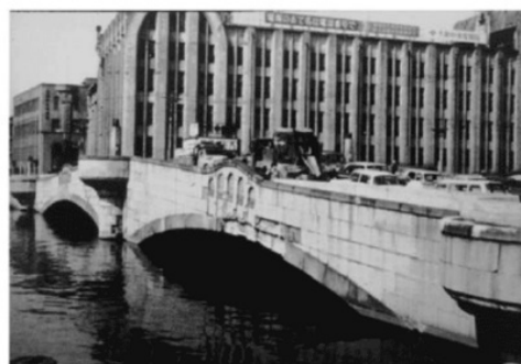
Figure 2.4 Subsidence of Bridges in Osaka City
