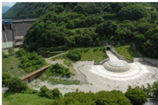
Sediment bypass facility
