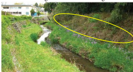
Thirteen years after construction: the natural connection between slope and river is maintained.
