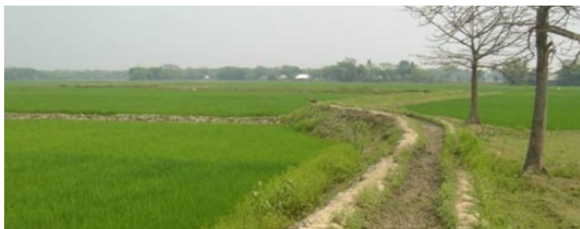
Figure 2.12 A Submerged Levee Protects Rice from Flooding (Haor District, Bangladesh)
