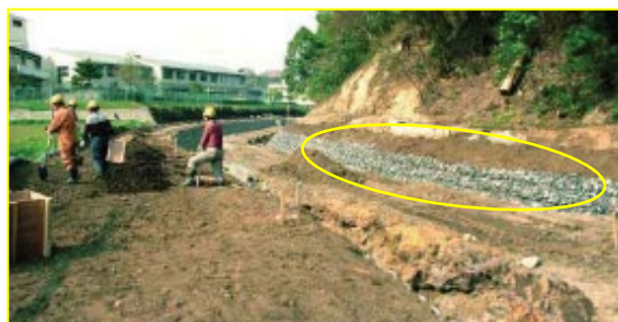
Renovation: gabion revetment on right bank
