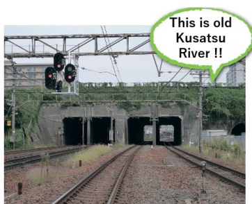
View of point 1 from the ground
