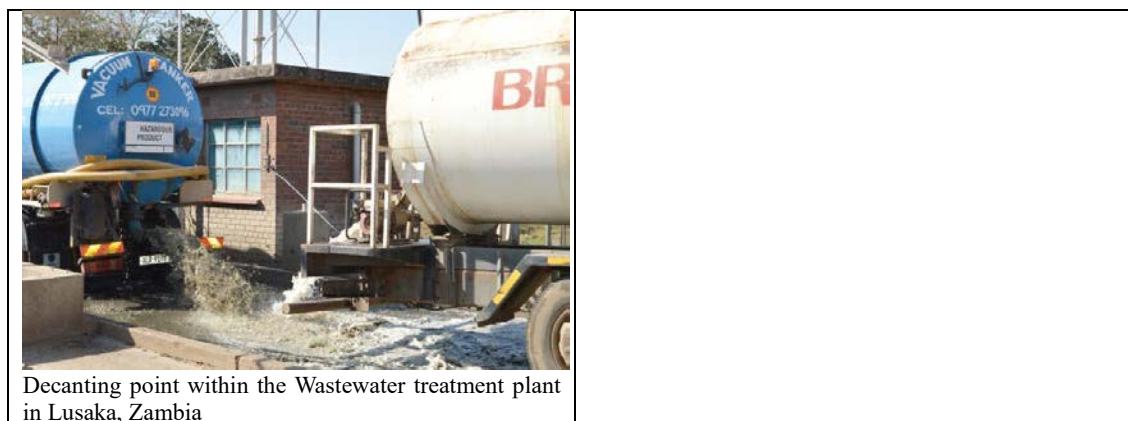
Figure 5-15 Sludge Discharge at Wastewater Treatment Plants
