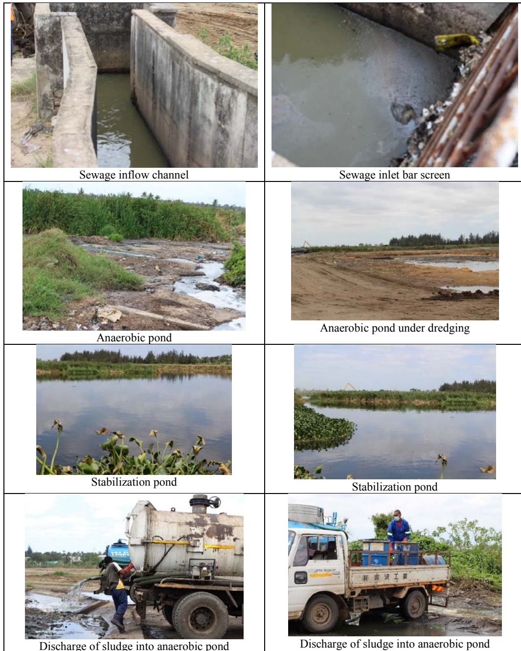
Figure 5-8 Situation of Existing Facilities in Infulene WWTP, Maputo, Mozambique
