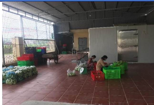
Upgrade of pre-processing house, Vinh Phuc cooperative (Vinh Phuc 12 th March 2020)
