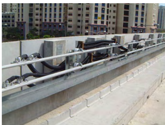
Figure 8-9: Power Rails
