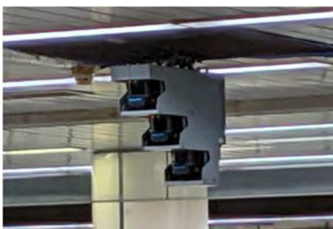
Figure 8-13: Train Automatic Stop-Position System
