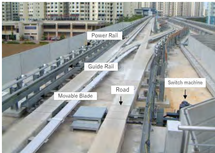
Figure 8-6: Appearance of the Track Course (Running Surface, Guide Rails, Switches)
