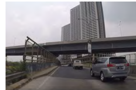
⑫ Road Bridge crossing Expressway and Viaduct of New Expressway
