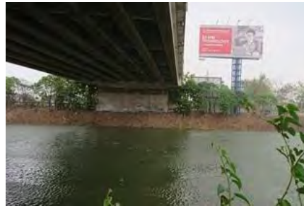
⑪ Road Bridge over a River
