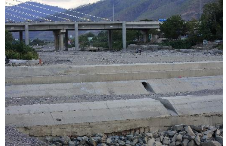
Downstream check dam
