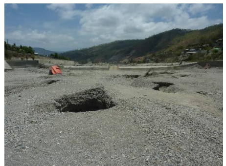
Upstream check dam
