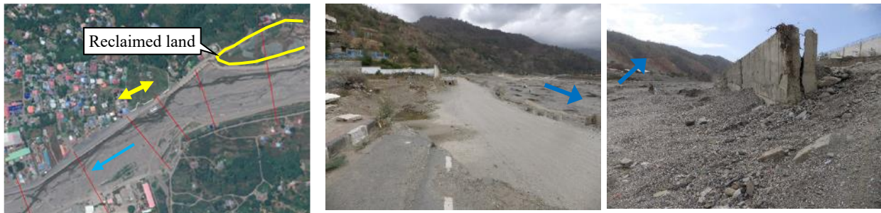
Figure 16 Damage to river wall (R7)
