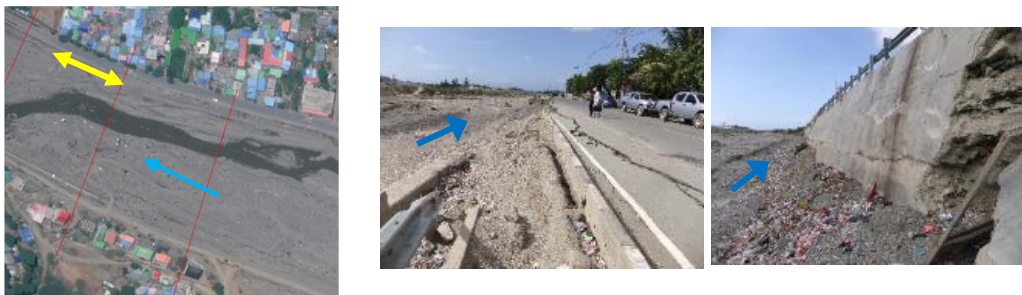
Figure 15 Damage to river wall (R6)
