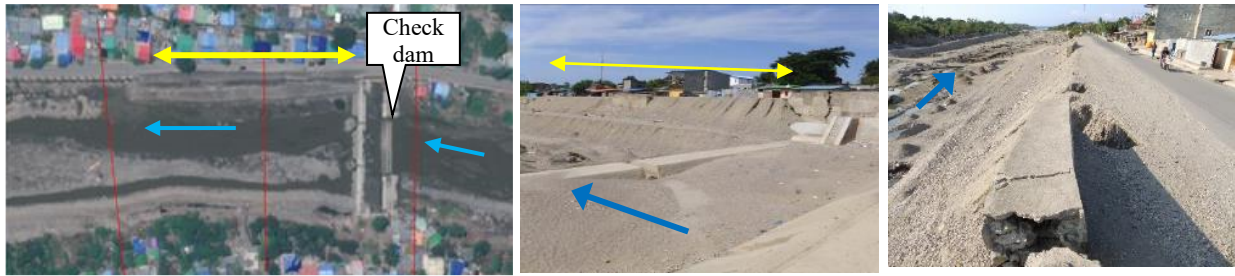
Figure 13 Damage to river wall (R4)
