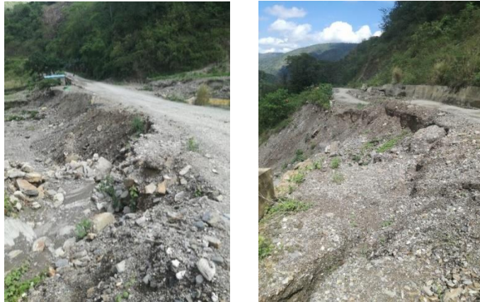
Figure 22 Cross culvert and road damage at 12.2 km (left) & Road damage at 15.4 km (right)
