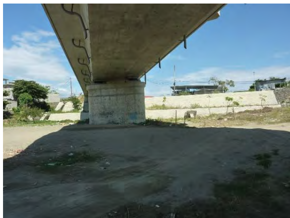
P5 橋脚と河川敷
