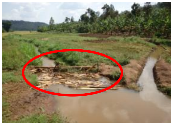
Photo-2 Drift wood branches on a simple diversion weir disturbs water flow in Gacenshero zone (Mushikiri Rice Growers Cooperative)
