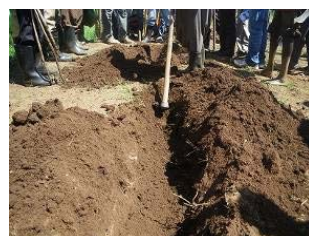
Making Ditch of 30cm Depth
