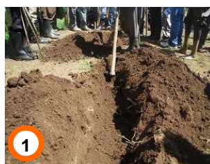
1 Making Ditch of 30cm Depth
