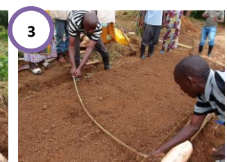
3 Leveling using a Wooden Pole
