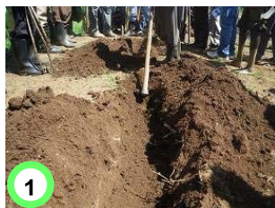
1 Making Ditch of 30cm Depth
