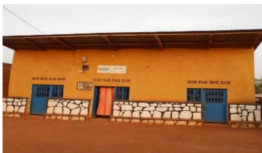
Photo 1 Constructed House for Business Expansion by Cooperative
