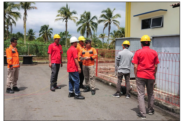
Staff engaged the maintenance at the Payakumbuh substations (West Sumatra)
