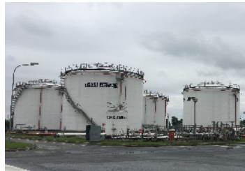
Aircraft Fuel Hydrant System Facility
