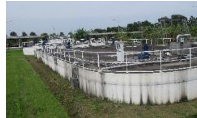
Sewerage Treatment Plant Facility
