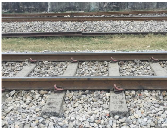
Roadbed Developed through the Project
