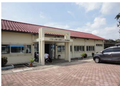
Exterior of Dumai VTS Center Building
