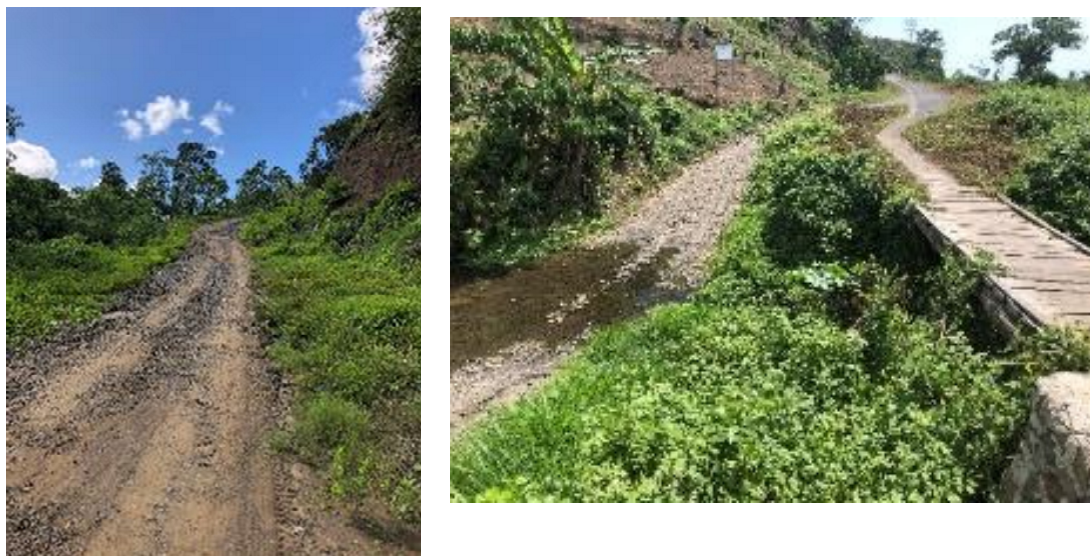
Unpaved Sector and Small Bridge Construction Site
