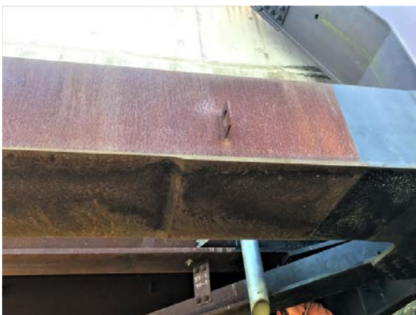
Weather-resistant steel (the right-hand side is painted for aesthetic purposes)
