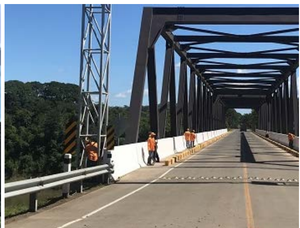
Regular maintenance work in progress
