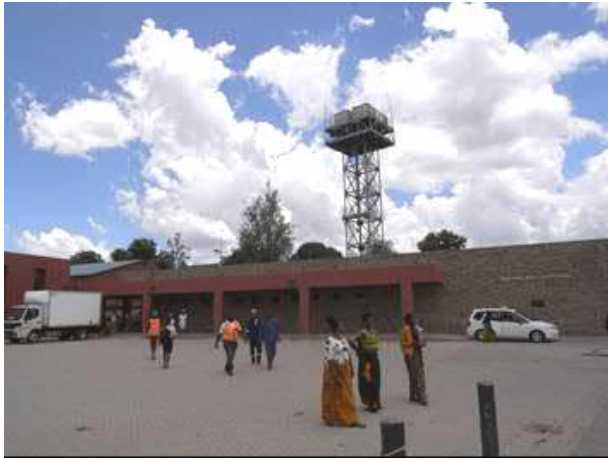
External appearance (main entrance)
