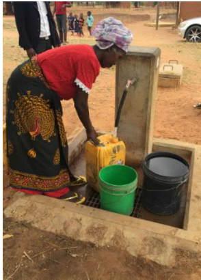
Level 2 water supply facility (Tabora municipality)
