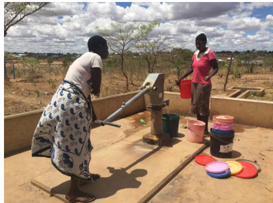
Level 1 water supply facility (Sikonge district)
