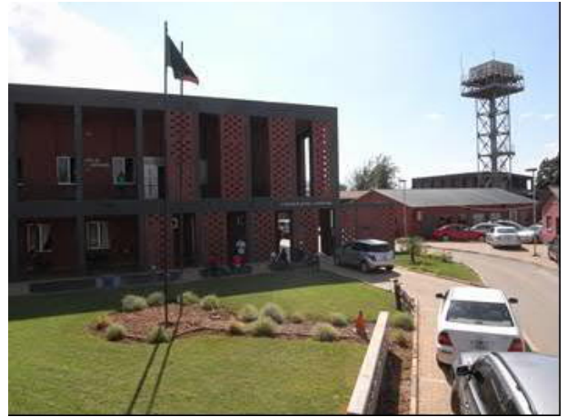
External appearance (main entrance)
