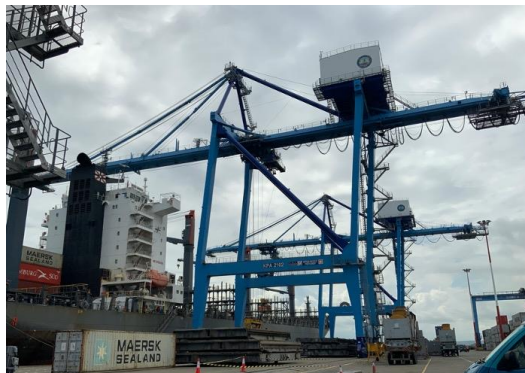
Berth 21 and SSGs built/procured in the project
