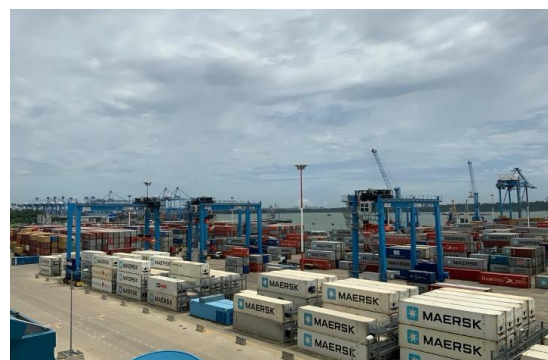
Newly constructed Container Terminal 2
