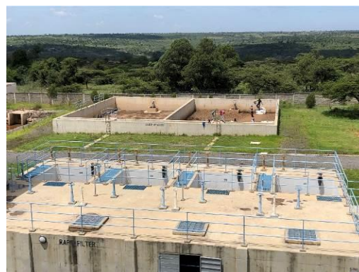
Newly constructed NWTP (front: rapid filter, back: sludge drying bed)
