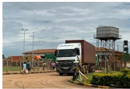
One of the border facilities assisted by a JICA technical cooperation project: Busia OSBP at the Kenya-Uganda border along the Northern Corridor
