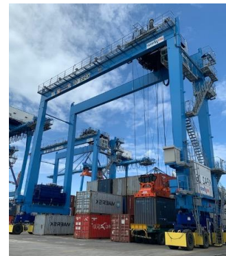
Container yard and RTGs constructed/procured in the project
