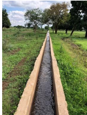
Canal developed by the project
