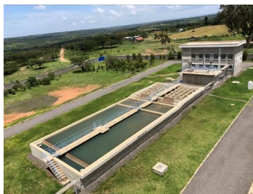
Newly constructed North Water Treatment Plant
