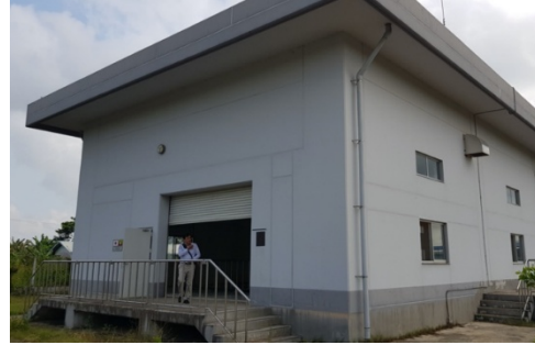
Pump House (at the time of ex-post evaluation)
