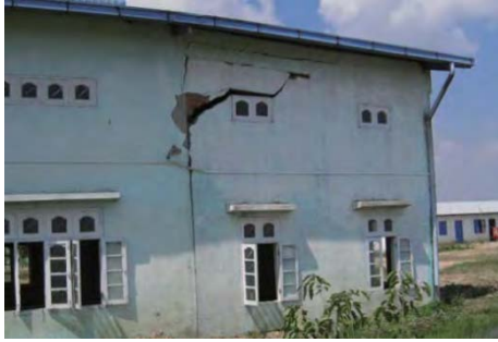
Pump House (at the time of planning)
