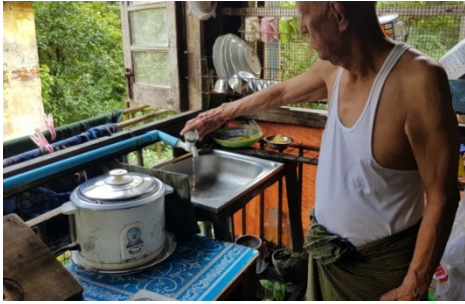
Water supply line installed in a house in Yankin Township
