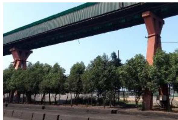
Tree planting near a conveyor
