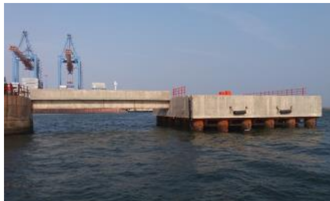
Mooring dolphin constructed by this project
