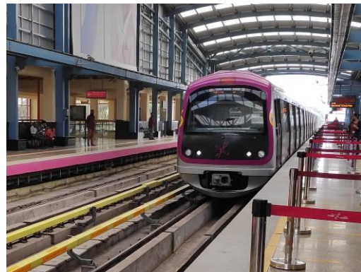
East-West line of Bangalore Metro constructed by the project
