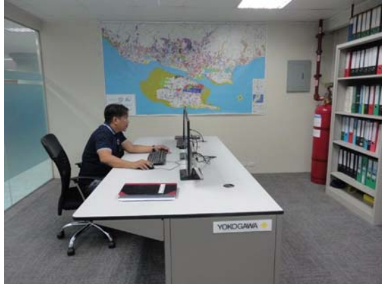
SCADA Room inside the MCWD Main Office
