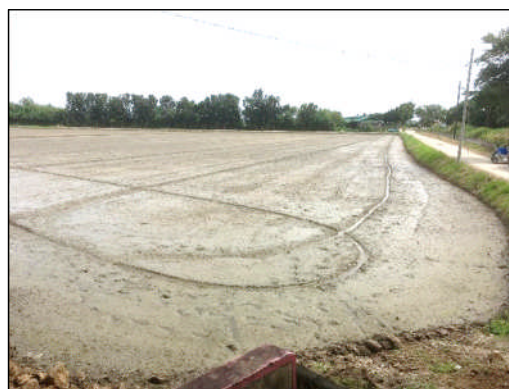
Communal Irrigation Facilities Constructed by This Project/Rice Field (Pampanga Province)
