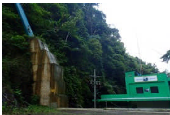
Photo 2: New and Renewable Energy Sector Hydroelectric Power Station (Laguna, Luzon Area)
