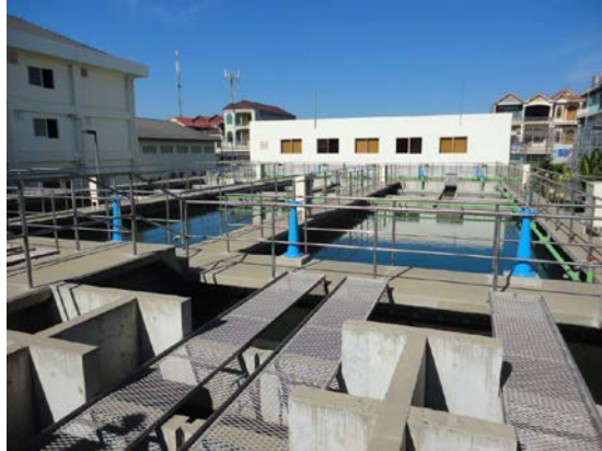
Flocculation Basin (front) and Sedimentation Basin (back) (Kampong Cham)
