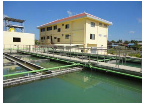
Sedimentation Basin and Administration Building (Battambang)
