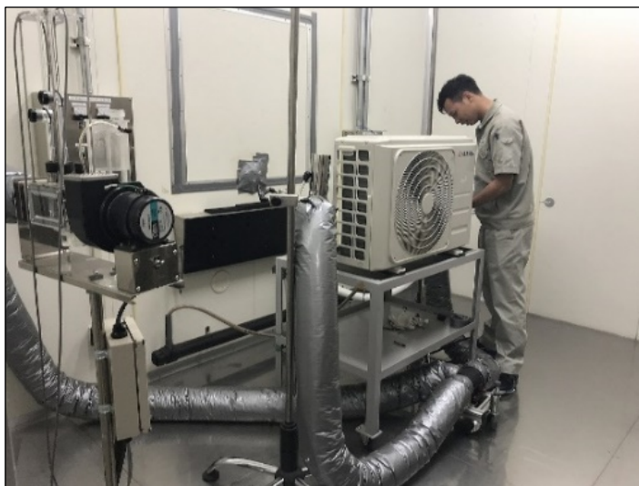
Testing equipment of the air conditioner provided by the project
